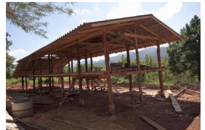
The new house under construction
